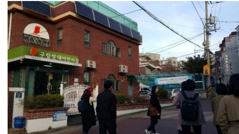
Daycare Center (Solar Panel)
