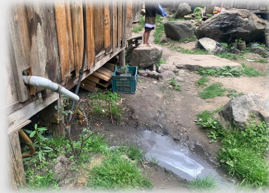
Waste water discharge from households at location 1
