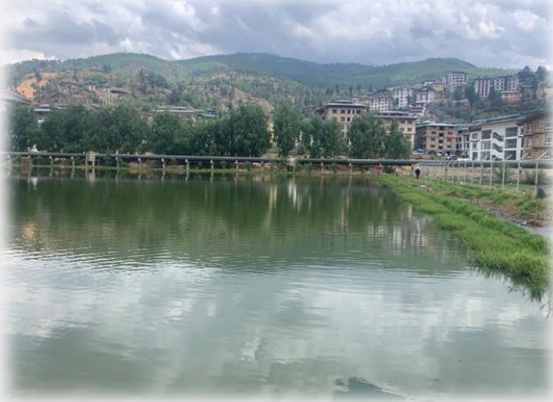
1.75 MLD WWTP during in Location 2, Babesa
